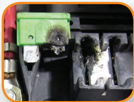
OE Unit is Prone to Melting and Heat Failure
